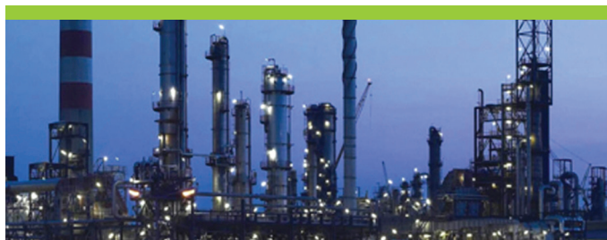
petrochina (refinery) Chengdu (China) - 60,000 m 3 /d
