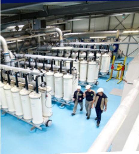
SUEZ provides a pre-treatment system, reverse osmosis desalination system, RO concentrate evaporation, together with a drying system and deep desalination system, through mixed-bed ion exchange for RO permeate, to remove nitrogen and phosphorus and ultimately achieve zero discharge. Every year, 15 tonnes of phosphorus discharge is avoided, and 230 tonnes of solid waste is reduced.
