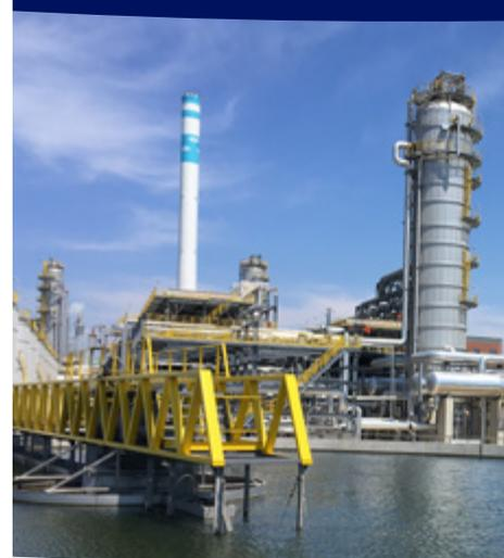
SUEZ provides treatment process design, Densadeg® pre-treatment system equipment and technical services for a mining wastewater treatment plant in Xi'an, which can significantly reduce contents of silicon and solid suspensions as well as total hardness in wastewater. By ensuring the subsequent stable operation of the membrane system as well as the evaporation system, zero discharge can thus be achieved.
