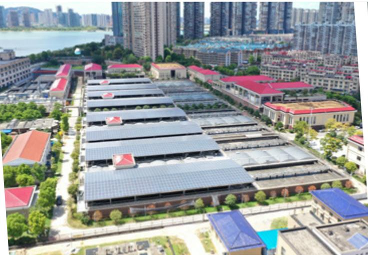
SUEZ recently signed a contract with Hunan Xinyuan Co., Ltd. to provide the AQUADVANCED® Plant solution to improve the plant's wastewater treatment performance. The plant's treatment capacity is 250,000 m<sup>3</sup>/day and the effluent will comply with Surface Water Class IV Standards. SUEZ will also provide a precision aeration system, which will cut energy consumption by 7%.
